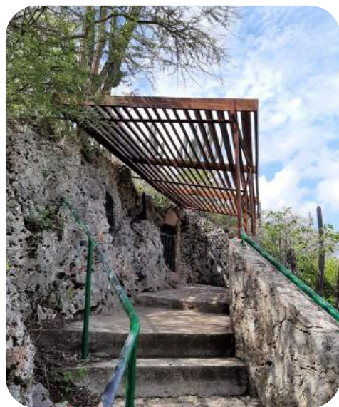
The new roof at the entrance of the Hato Caves
