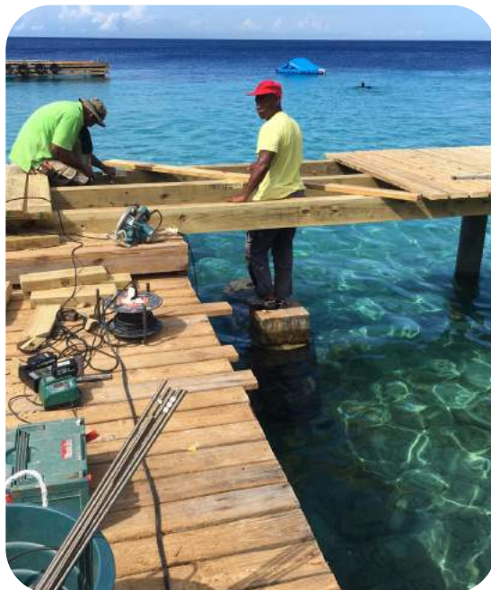
It took the workers a full week to renew the pier
