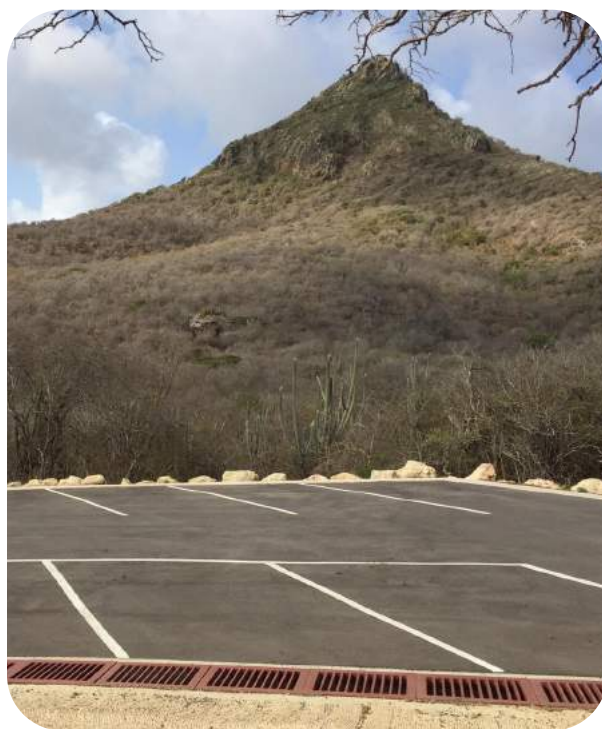
Asphalted the parking lot at the foot of the Christoffel Mountain
