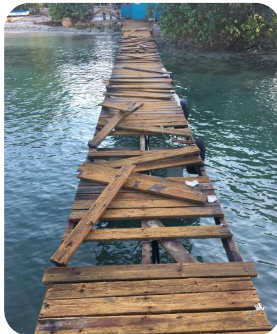
All the planks got washed away by the storm
